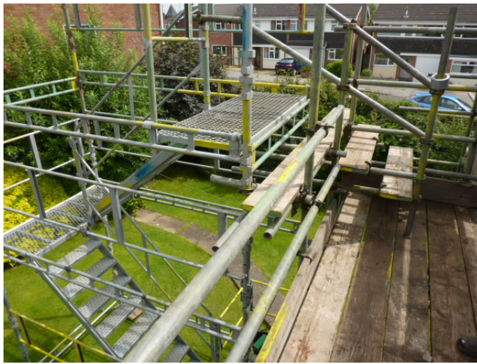
Photo 4: Examples of sealing of full enclosure around gutter and pipework
